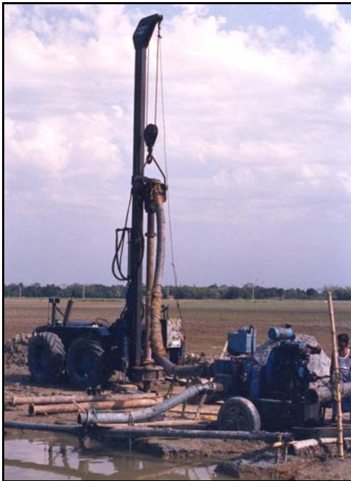
Figure 7 Reverse-circulation drilling rig
