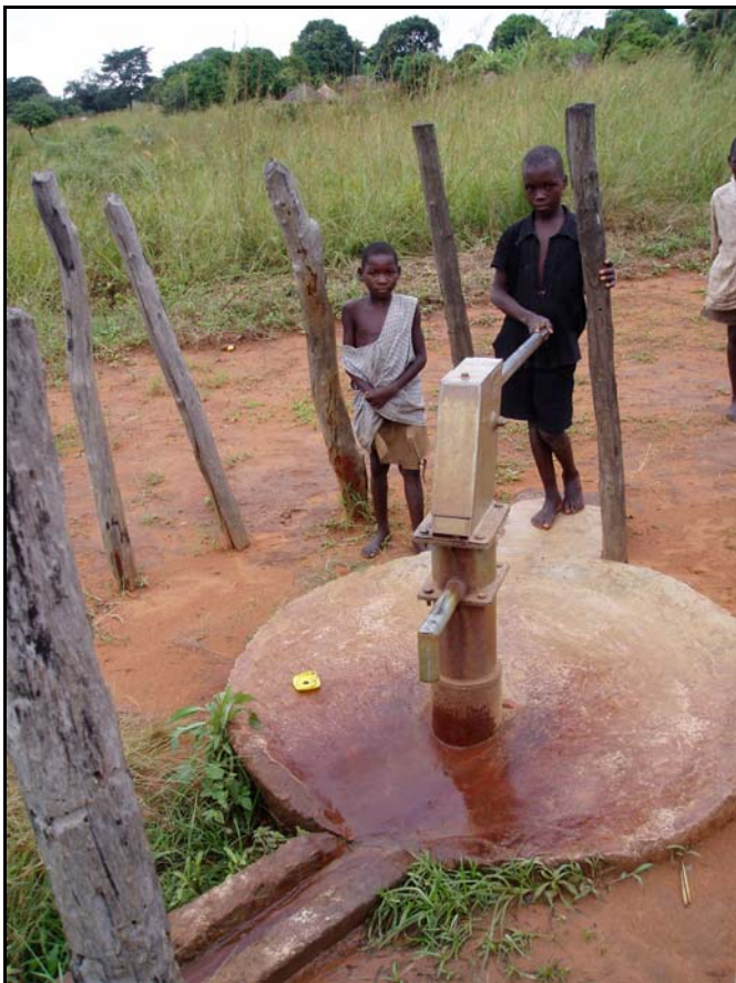
Iron-rich groundwater causing iron staining at a handpump
