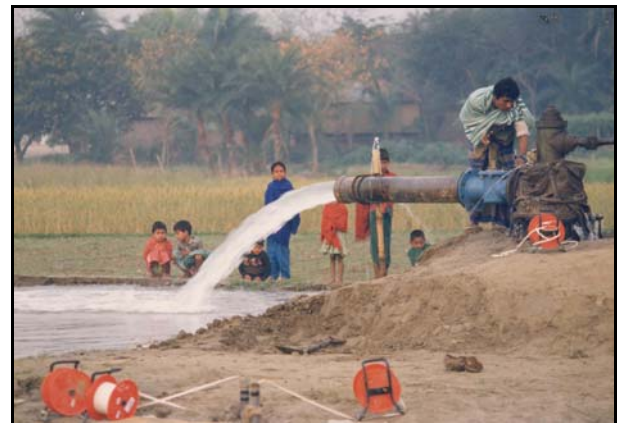
Figure 6 High yielding irrigation tubewell, with monitoring piezometers in the foreground
