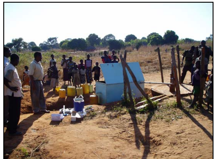
The same borehole after iron filter installation
