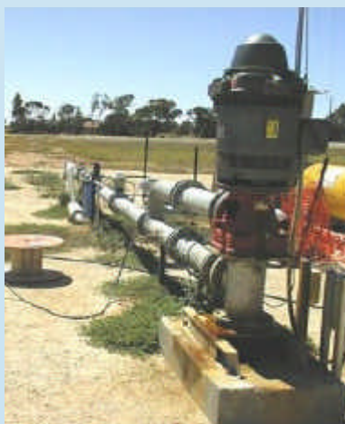
Under some conditions reclaimed water can be injected into a confined brackish aquifer and stored for subsequent irrigation supplies. An example in Australia.
