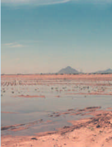
Large spreading basins are used to recharge water near Phoenix, Arizona. The water is imported by aquaduct.
